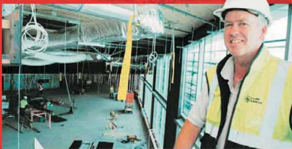
Surveyor Mike Wilson laid out the architectural services boxes that run the length of the ceiling in Air NZ's new Koru Lounge.
