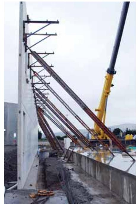
*It was a technical job to prop up large precast panels used to build the new facility at the Christchurch wastewater treatment plant.*
