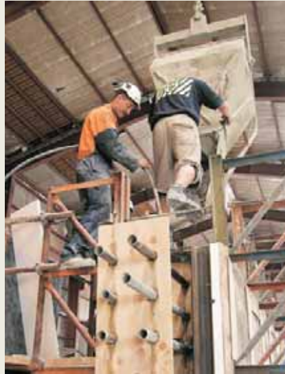
The precast team pours concrete into a form.
