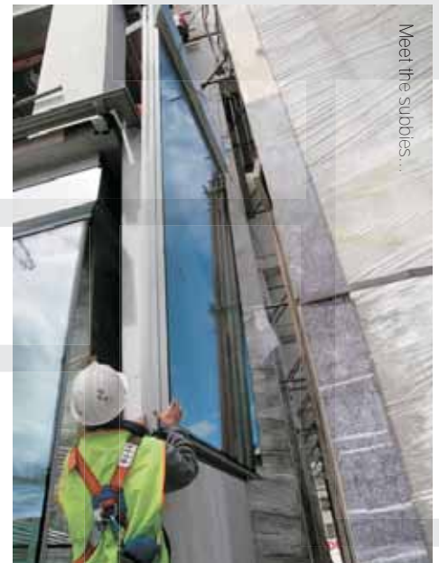
The Thermosash crew install a double-glazed glass wall unit.
