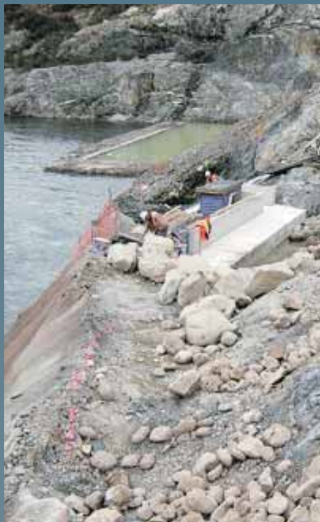
The Opuha Dam project was tough work in tough conditions.
