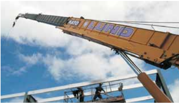
At work on the new warehouse for Canterbury Wool Scourers.
