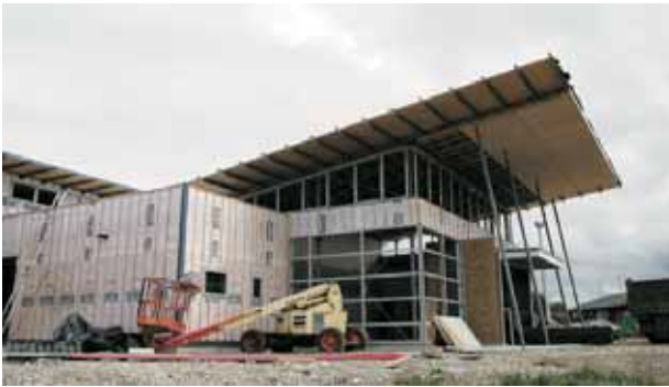
The T-TEC building in Timaru.
